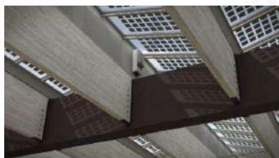
Rotterdam Railway Station Photo: Scheuten Solar
