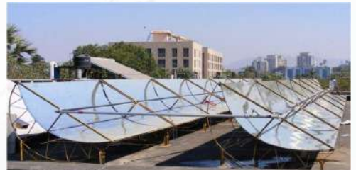
S. Panse, Compound Parabolic Solar Collectors for Process Heat
